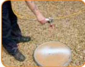
**2.** Point the nozzle at the area you wish to protect and hold the spray gun 12-15 inches from the substrate. Use a shield to prevent overspray.
