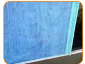
**5.** Leave to dry in a rain free environment and allow 2 hours at room temperature to dry. The product will gain maximum strength after 3 days.
