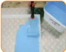
**1.** Once you have masked off the area, apply a base coat of Skudo to the substrate paying particular attention to vulnerable areas such as corners. Allow to dry for 15 minutes or until coating is tacky.
