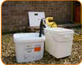
**1.** You need to purge the spray equipment before you begin application. First place the inlet suction hose into the Skudo container and purge the airless spray pump with material. Then purge the airless spray gun and test the spray pattern.
