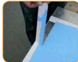
**4.** Remove the masking tape while the product is still wet. This helps to achieve a good thick edge that is easier to peel when the product is no longer required.
