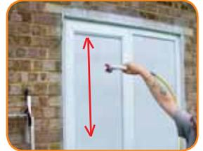
**5.** When the surface is fully covered, repeat with the spray process in a vertical direction. Take care to ensure that corners and inside edges are coated thoroughly. If the coating is too thin in these areas it may become difficult to remove.
